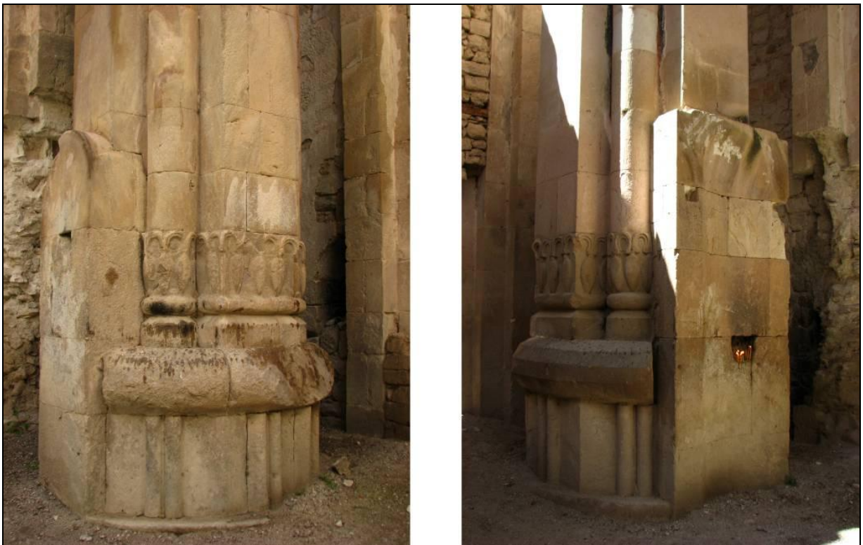
Fig. 7. Ishkhani Chathedral. Interior. Niches in the north-west and south-west piers of the dome
